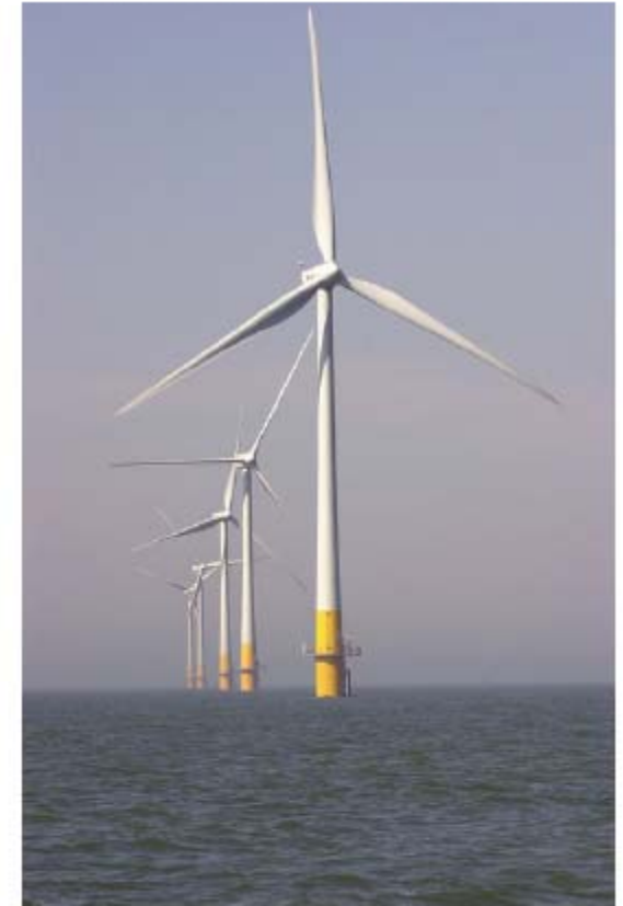
Figure 10.1. Kentish Flats – a shallow offshore wind farm. Each rotor has a diameter of 90 m centred on a hub height of 70 m. Each “3 MW” turbine weighs 500 tons, half of which is its foundation.
