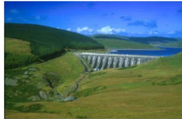
Figure 8.1. Nant-y-Moch dam, part of a 55 MW hydroelectric scheme in Wales. Photo by Dave Newbould, www.origins-photography.co.uk .
